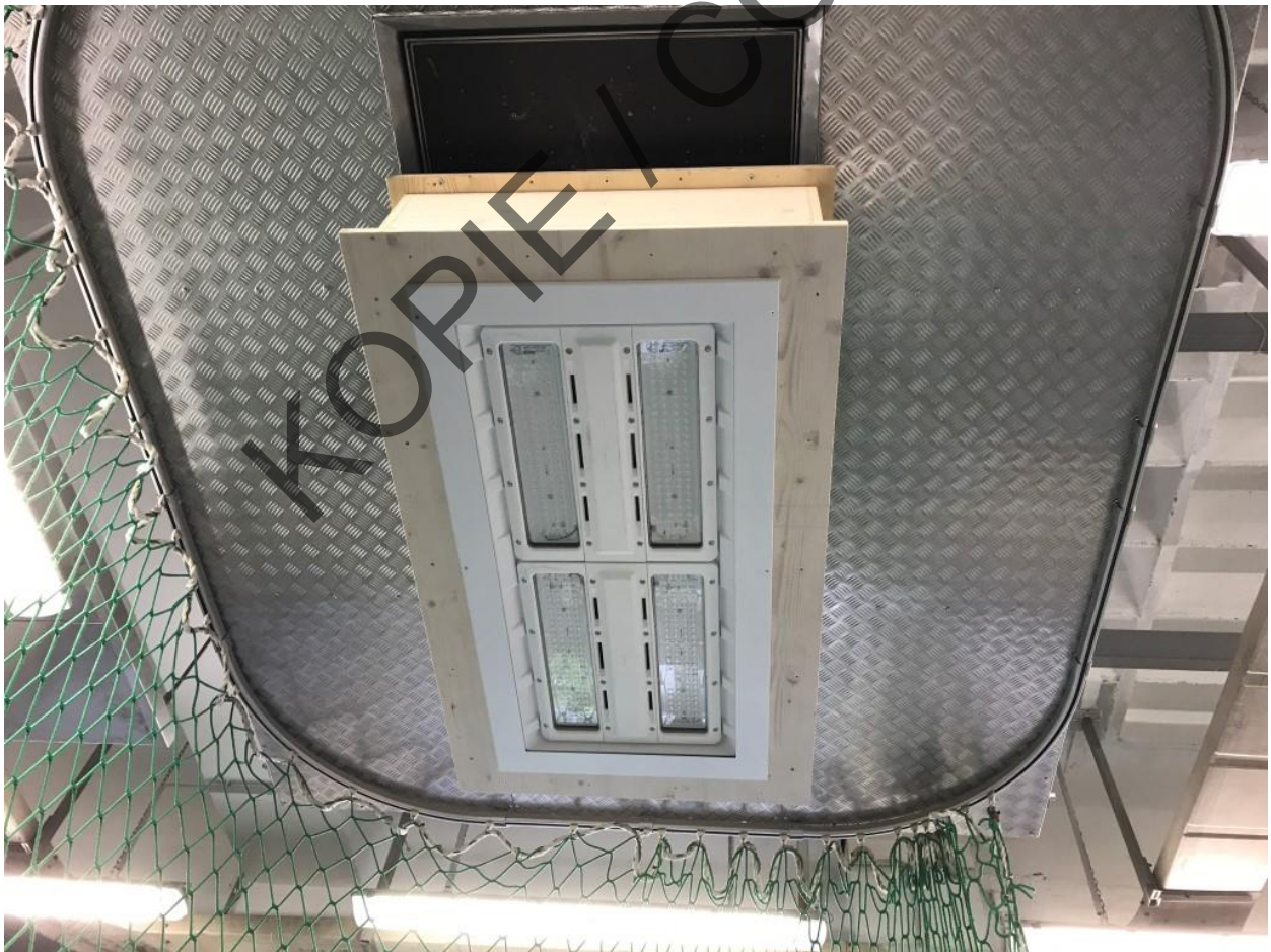
Picture 4: CR L35k-840 PC WB LDO WH – recessed in ceiling
